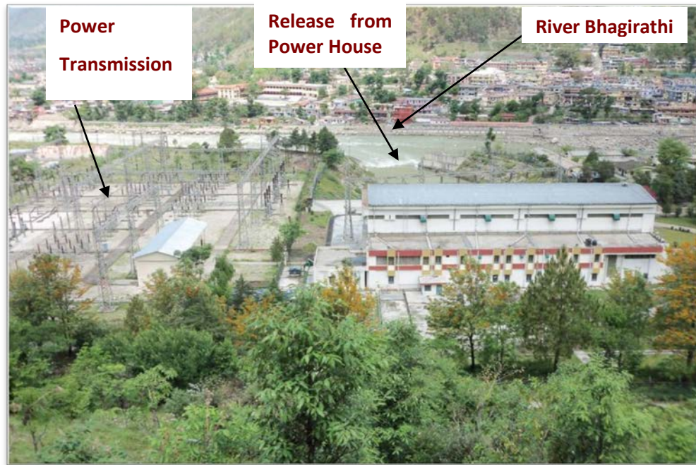
Plate 2.1: Photograph Showing Merging of Water Released after Power Generation with River Bhagirathi at Maneri-Bhali I HEP along with Power House and Transmission Lines
